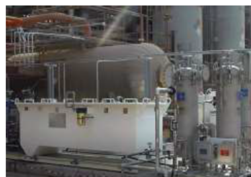
MAS Unit with Visual Oily-Fluid Breakthrough Indicator (VOBI)
