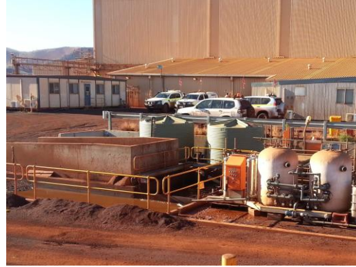
The mine site collection sump with evident detergent clearly visible & Filter system as installed
