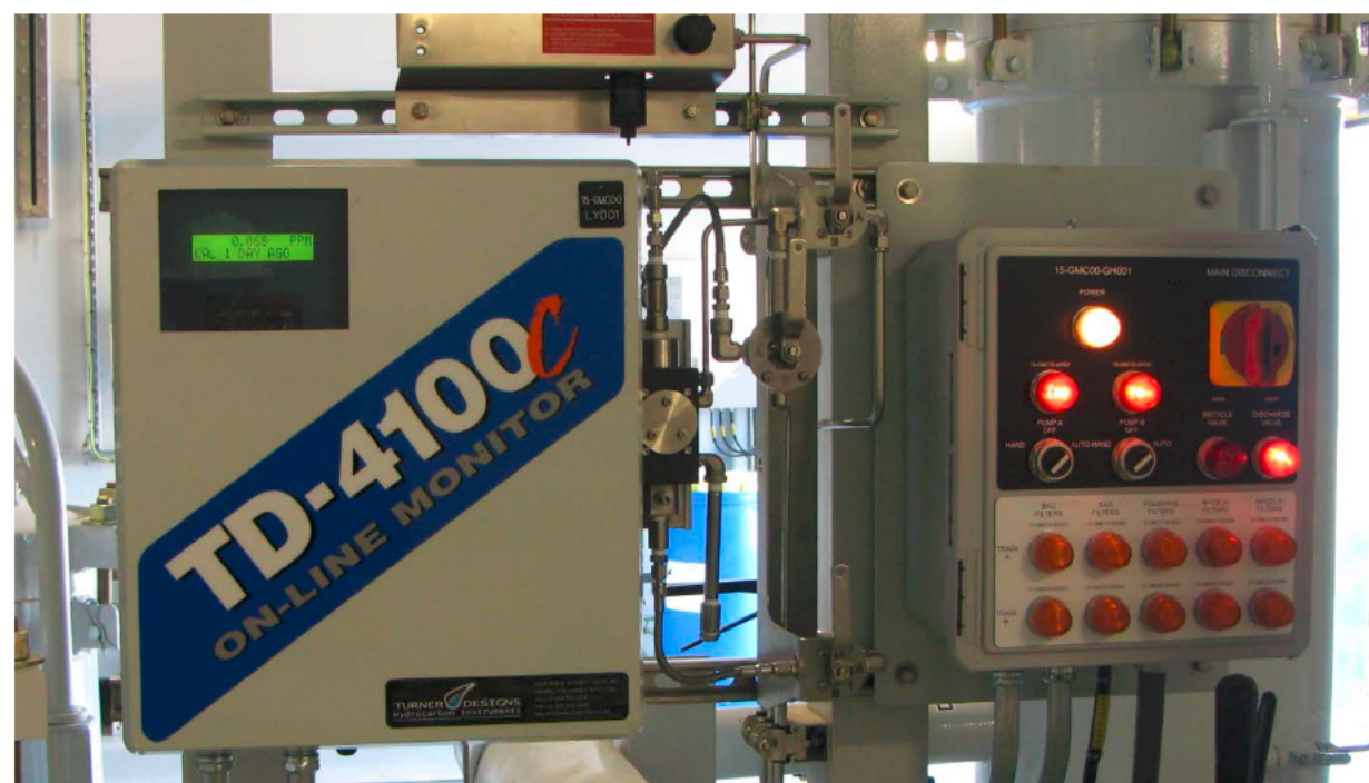
Integrated controls with on-line oil in water monitor. Note discharge level shown – 0.068 ppm or 68 ppb.
