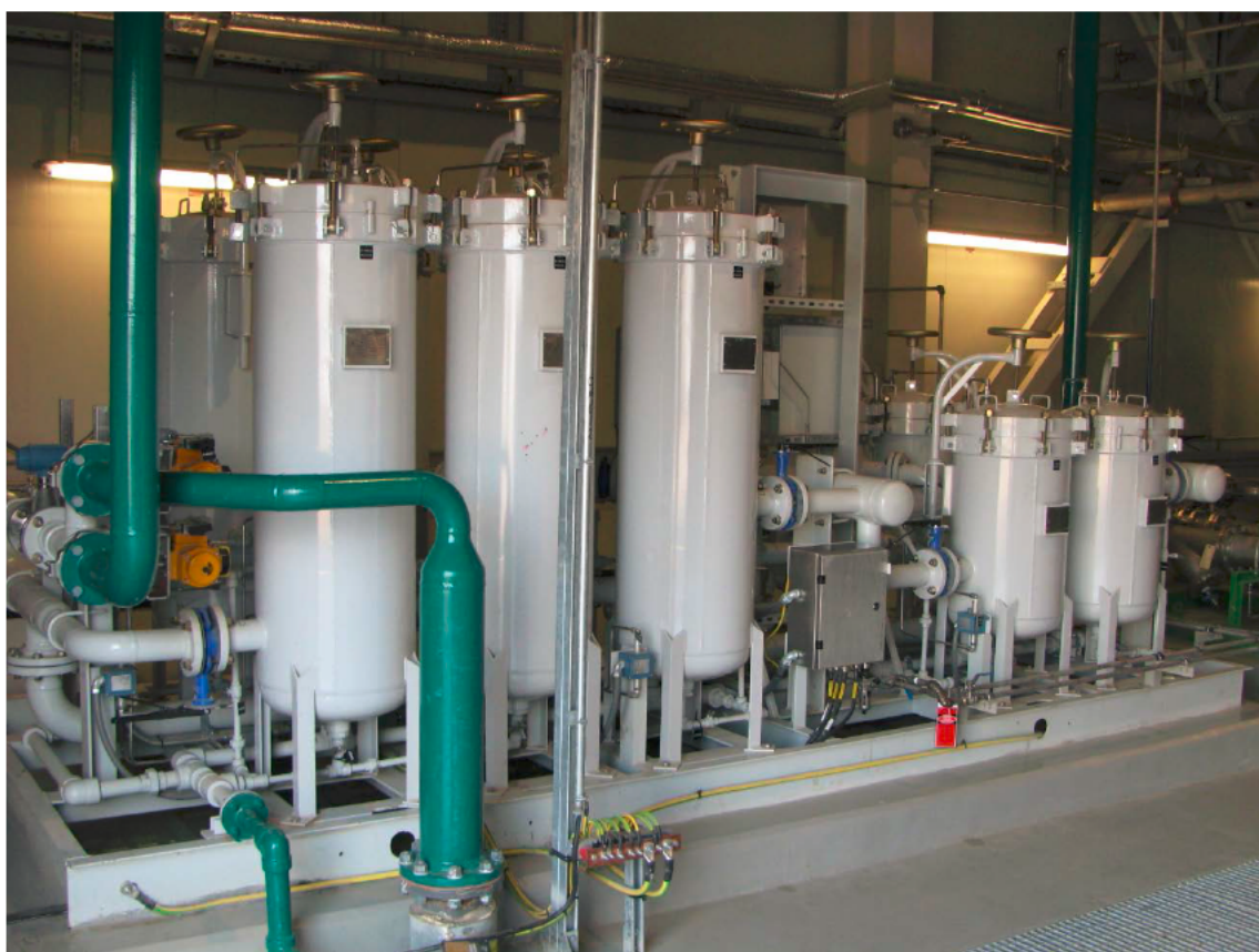
5 stage filtration with redundancy for complete oil removal
