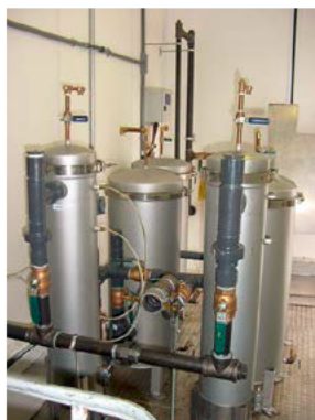
Bag Filter and Polisher System
